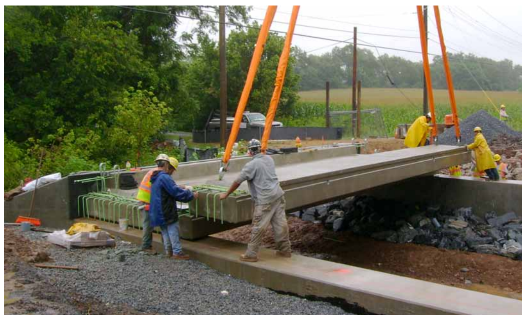
Precast slabs and other innovations helped the Maryland SHA cut construction time and enhance quality on a bridge replacement project.
