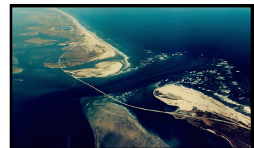
Figure 2—Aerial photo of Bonner Bridge
