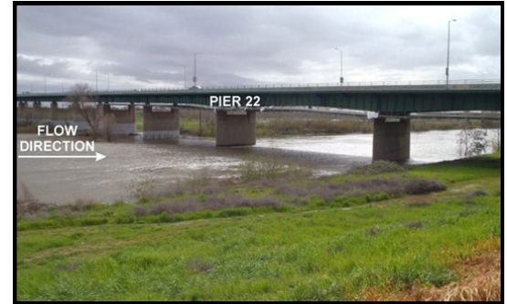
Figure 3— Feather River Bridge: Br. No. 18-0009 in Sutter County, CA
