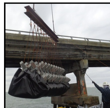
Figure 18—Geotextile Filter Applied to A-jack® Logs
