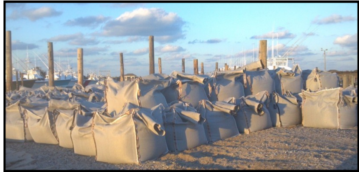
Figure 11—Geotextile Sand Bag Stockpile (4'x4'x4' cubes)
