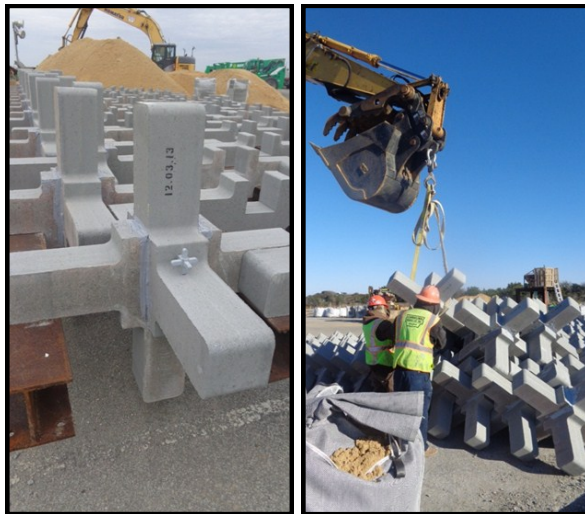
Figure 15—A-jacks® Assembly Area and Stockpile
