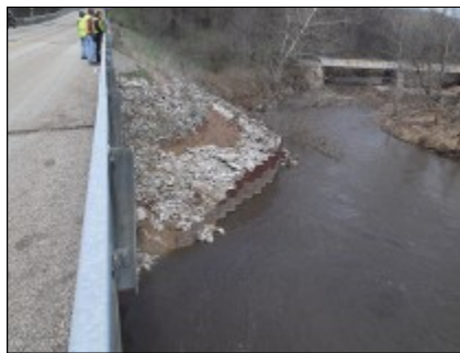
View of Upstream Abutment Cone
