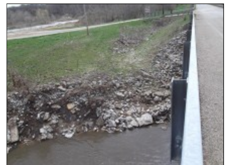
View of Upstream Face Outside Bend
