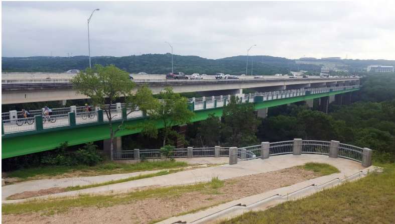
Figure 1: Mopac Mobility Bridges. (Image courtesy of the city of Austin)
