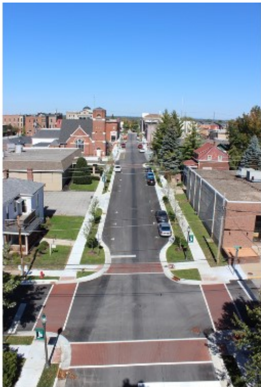
Figure 1: City of Greencastle streetscape improvements. (Image courtesy of the city of Greencastle Mayor's Office)
