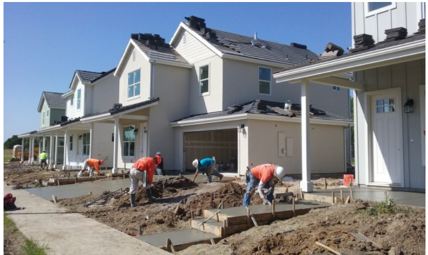
Figure 6: Construction on affordable homes for sale in the Promise Zone. (Image courtesy of Sacramento Housing and Redevelopment Agency)
