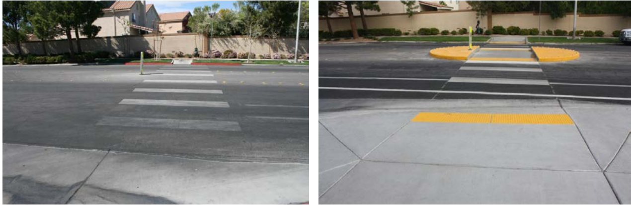
Figure 3: Piggott Elementary School crosswalk before (left) and after (right) school walk audit. (Image courtesy of City of Las Vegas)
