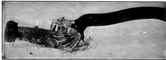
FIG. 64.—Effect of corrosion on battery cable terminals.
