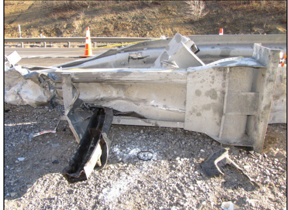
Figure 4: South-facing image depicting the choked end terminal and the bumper reinforcement beam.
