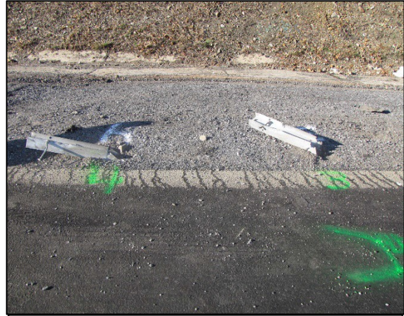
Figure 11: North-facing view of deformed Post 3 (right) and Post 4 (left).
