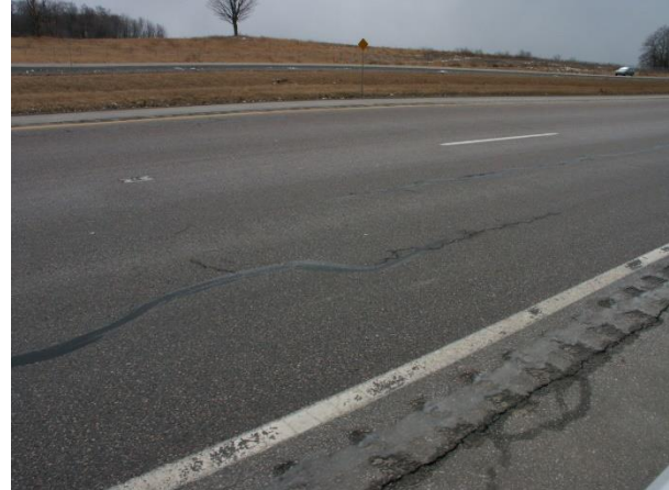
C. Second view of first stage—occurrence of short longitudinal cracks in and/or adjacent to the wheel path.
