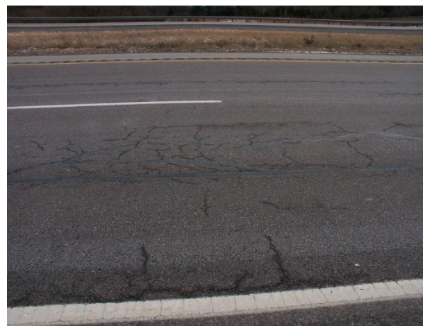
C. Second view of first stage—occurrence of short longitudinal cracks in and/or adjacent to the wheel path.
