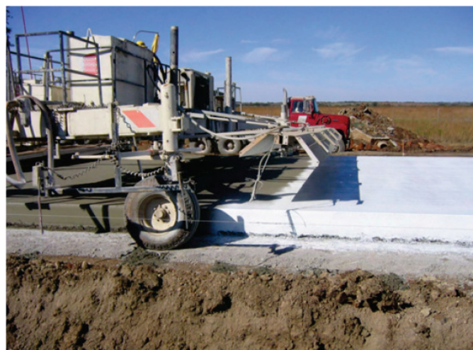
Figure 3. Spray equipment mounted on self-propelled unit applying curing compound to surface and sides of slipformed concrete pavement (Taylor et al. 2007).
