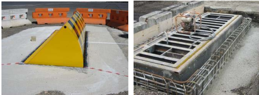
Figure 10. Photos. Examples of standard deep-foundation wedges.
