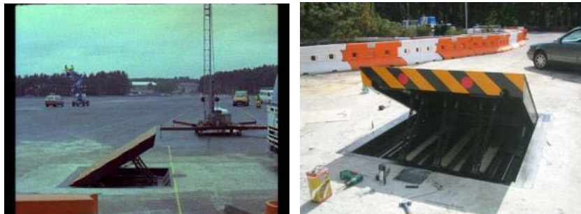
Figure 12. Photos. Examples of shallow-mounted wedges.
