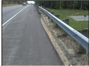
**Figure 2:** Orange paint marks show case vehicle's path toward first contact with west guardrail
