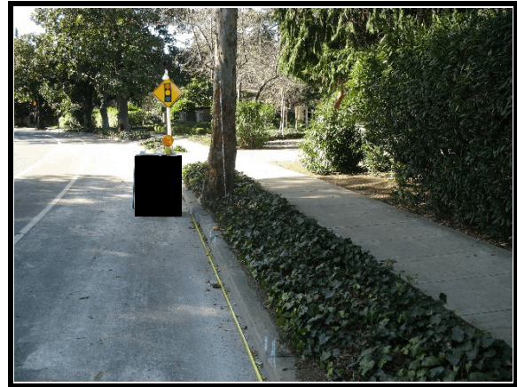
Figure 4. Area of impact with tree
