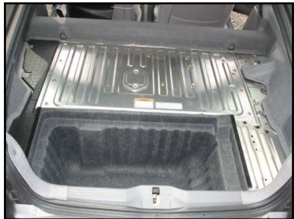
Figure 9: View of the battery compartment location.
