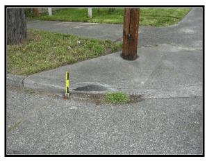
**Figure 4**. Contact to curb during rotation (area of trip)
