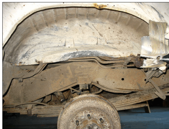
Figure 9: Black tire tread marks and abrasions on inside of Ford's left rear wheel well
