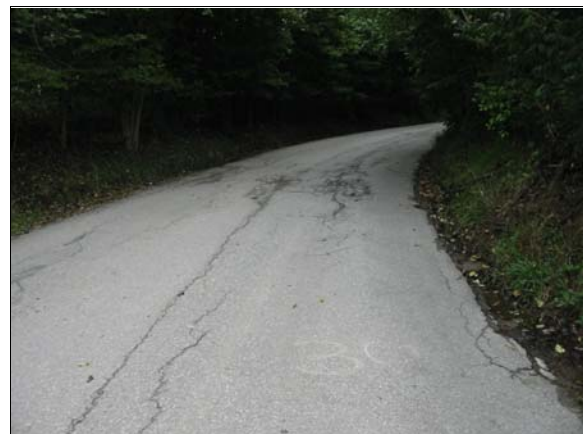
Figure 1: Approach of case vehicle westbound, approximately 30 meters (98 feet) from impact area
