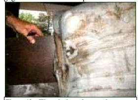
Figure 12. Water leakage from tank.
