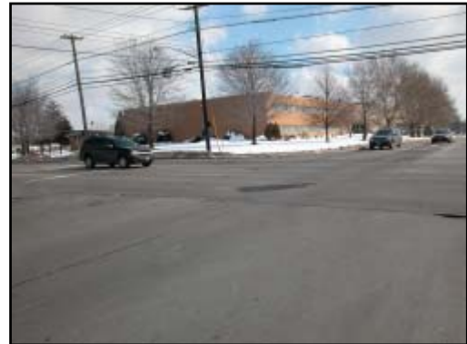
Figure 2. Northeast view of the intersection.
