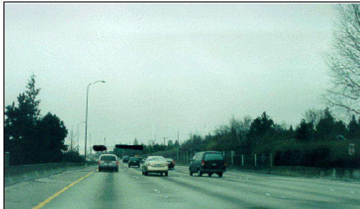
Figure 1. Area of POI, traveling south
